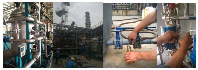
Left: Single housing 20 m3/hr treating Coker Process water in a refinery and installation Right: Taking raw water sample and permeate sample
